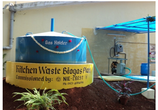
Kitchen waste Biogas Plant of 100 Kg/day implemented by NIE-CREST
